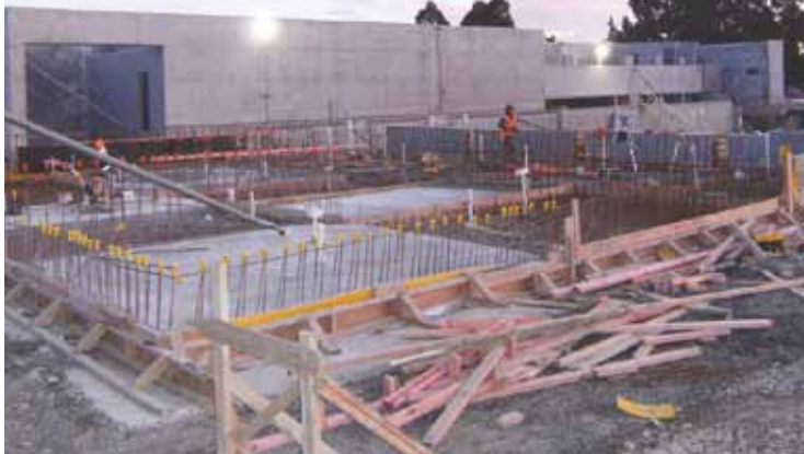
The leisure pool floor slabs are poured. The learners' pool panels are up (at right).
