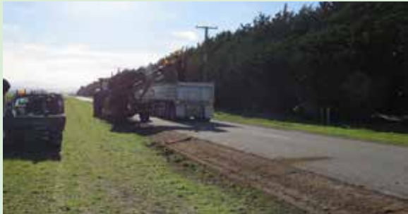
Shoulder removal underway along Te Pirita Road near Hororata
