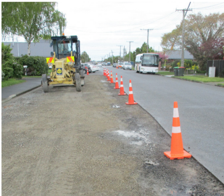
Work on the shoulder on West Belt, Lincoln being formed and sealed.
