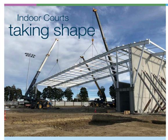
The Foster Park Indoor Courts have moved a step closer to being indoors with the first framing for the roof now in place.
