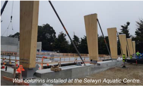
Wall columns installed at the Selwyn Aquatic Centre.
