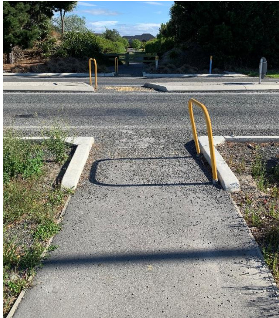
Photograph 3: Pedestrian Refuge Across SH73
