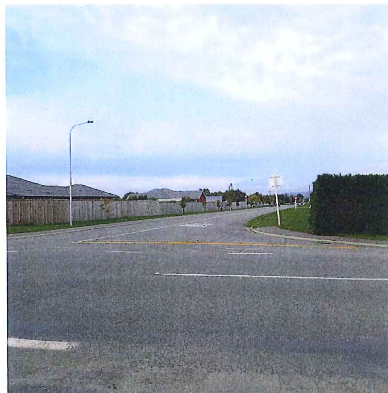
TRICES ROAD AT NW CORNER OF SITE
