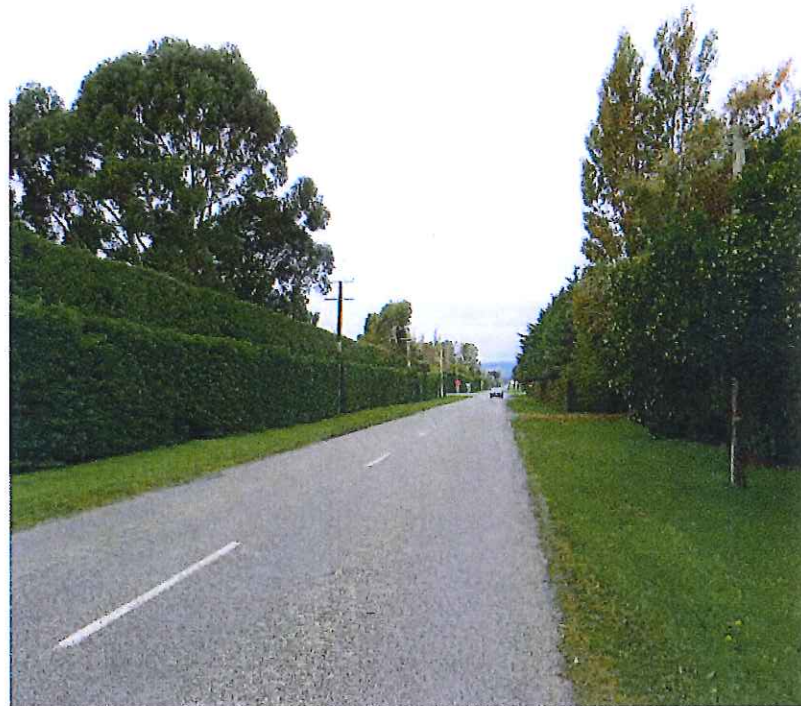
TRICES ROAD THRESHOLD EAST TOWARDS TOSWILL ROAD
