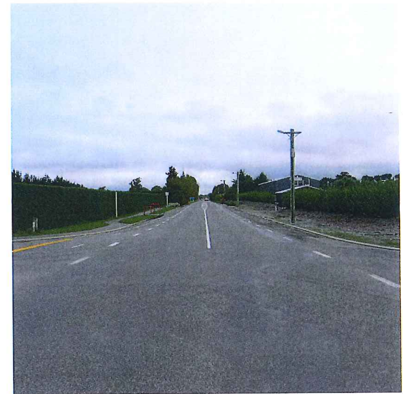
GATEWAY EXITING ALONG BIRCHS ROAD
