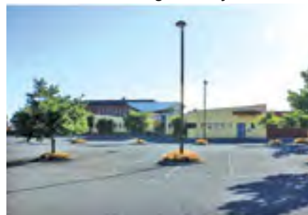
Rolleston Community Centre Source: Selwyn District Council
