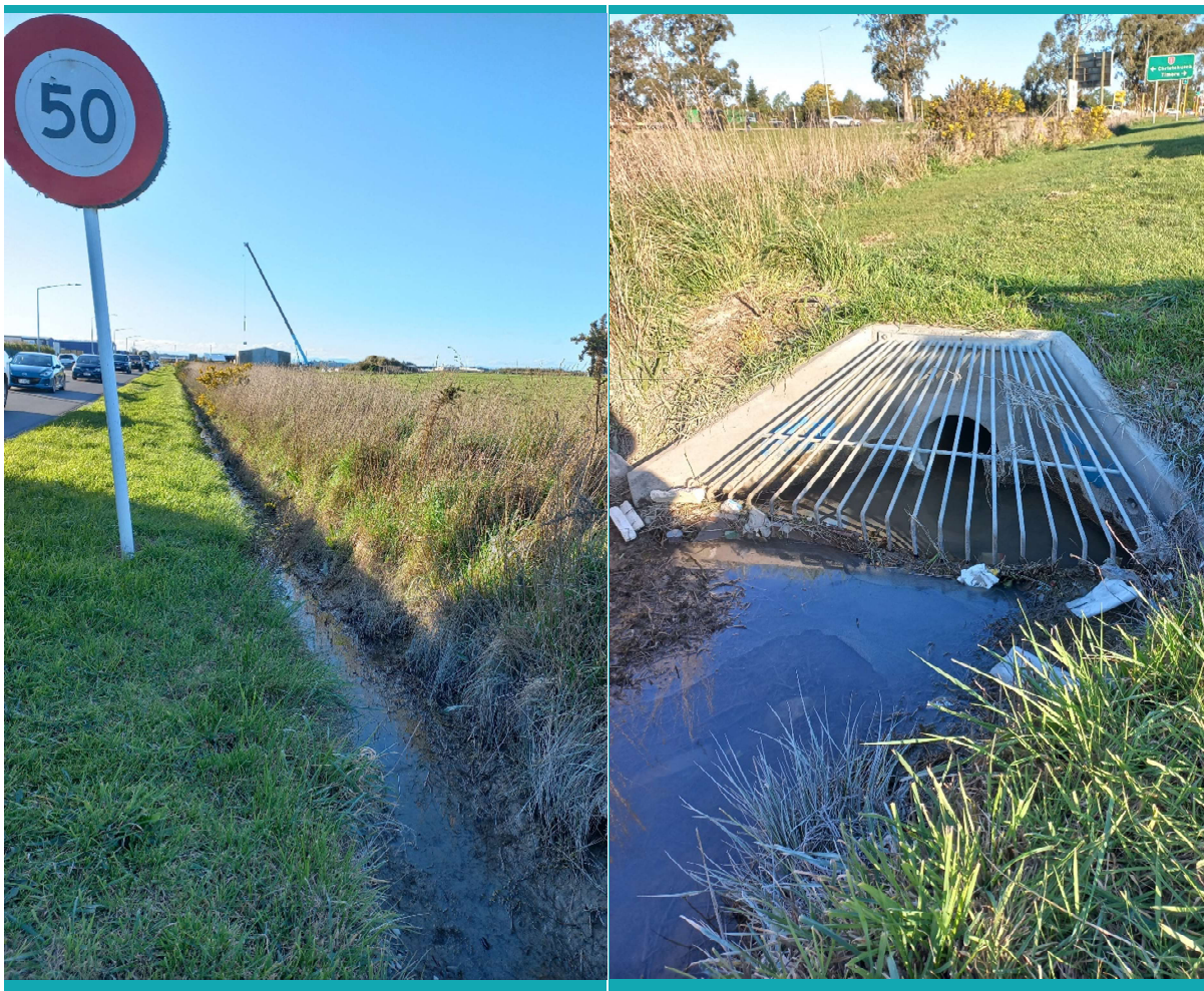
Figure 4. Images of the open drain (left) and entry to the culverted/piped section (right) of the stockwater race along Hoskyns Road.
