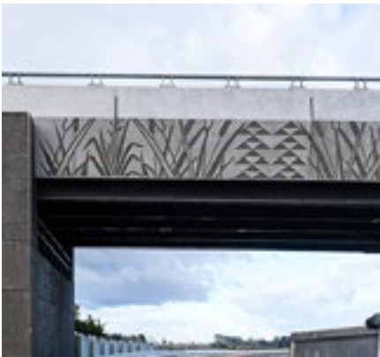
Precast concrete bridge barrier with pattern applied
