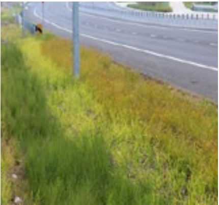
Planted verges / swales to reduce ongoing maintenance requirements
