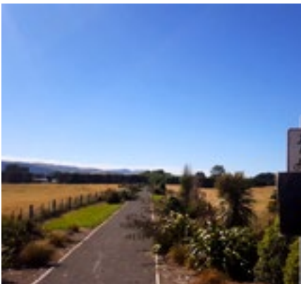
Off road asphalt shared path with native planted verges
