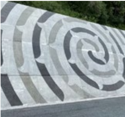
Concrete abutment walls, with vapor blasted patterns
