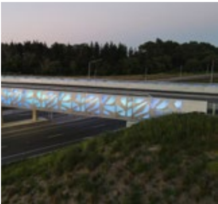
Steel shroud applied to bridge barrier
