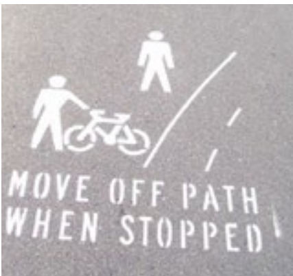
Example of surface markings that can be used to warn users of conflicts
