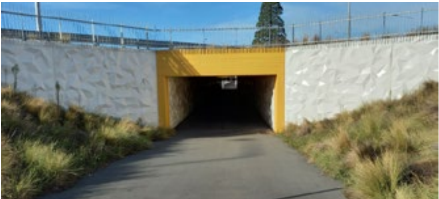
Example of subway entrance - treatments include low level planting, minimum clearance dimensions, pedestrian balustrades, clear sight lines and abutment wall patterning
