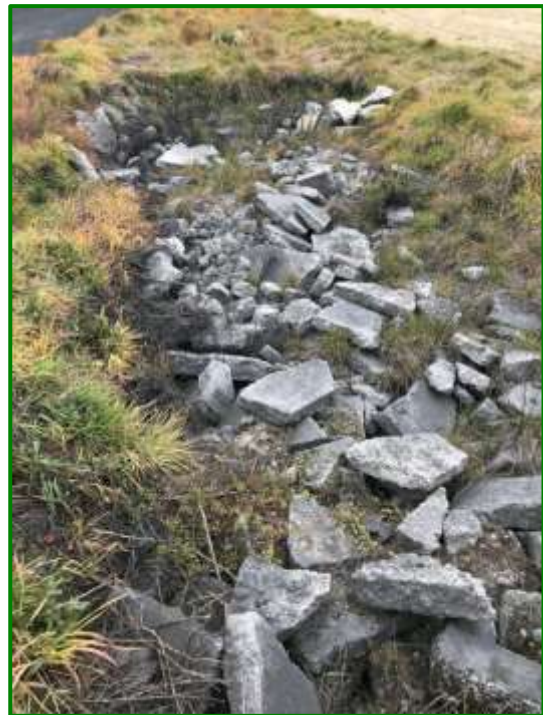
Photo 2: Soak pit filled with concrete
