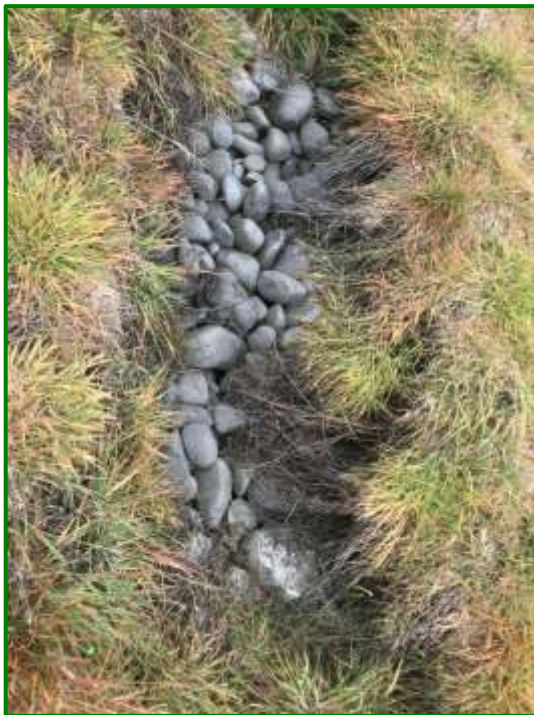
Photo 1: Soak pit filled with boulders
