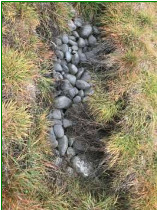
Photo 1: Soak pit filled with boulders
