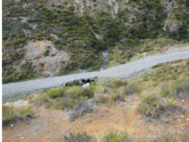
Photo 6: Culvert Across Existing Access Road
