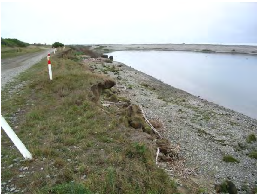
Photo 1: Access road erosion (taken April 2008)
