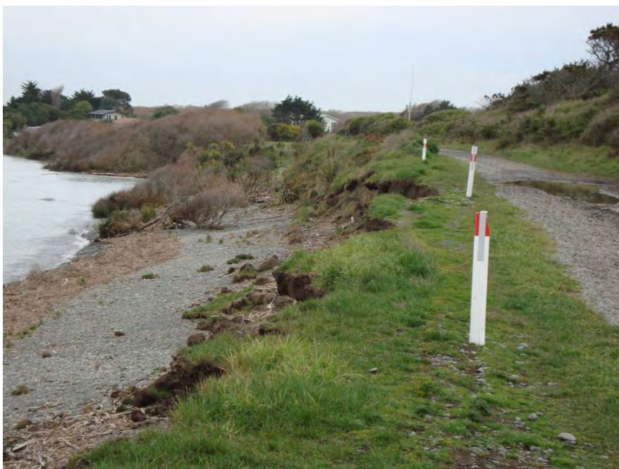
Photo 2: Access road erosion (taken September 2008)
