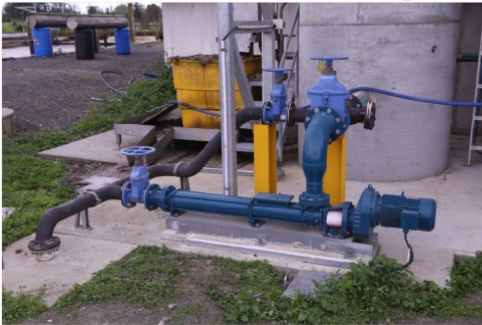
Figure 4-9 WAS Pump Station at Te Awamutu
