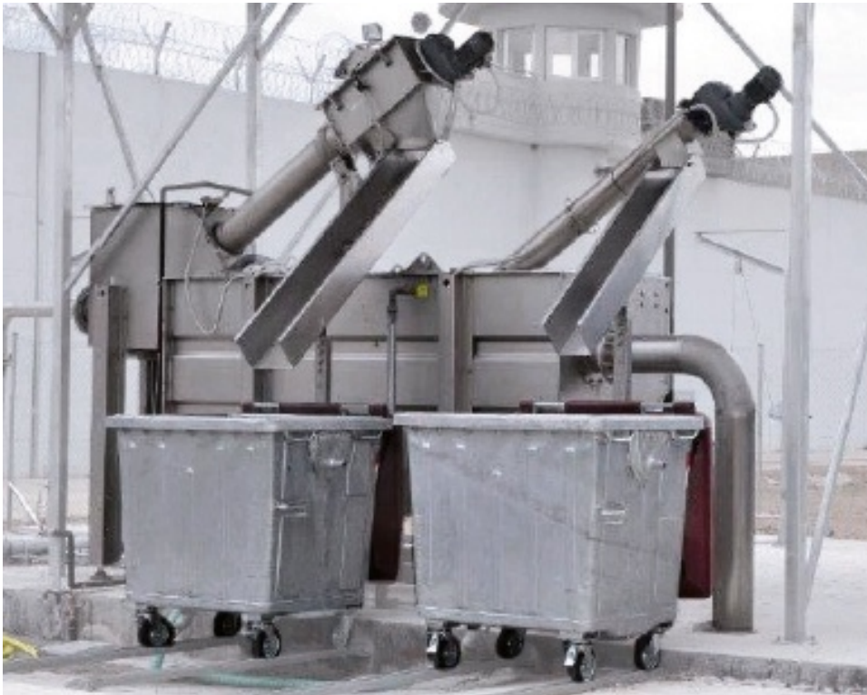
Figure 4-4 An example of an above ground combined inlet works installation
