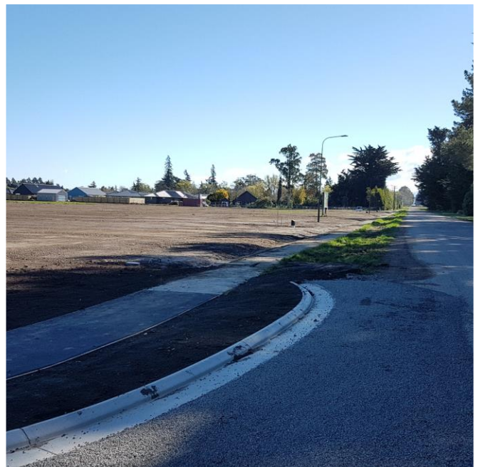
New kerbing and footpath (meeting the existing) and the lights installed along Hoskyns Road (towards Courtenay Road)
