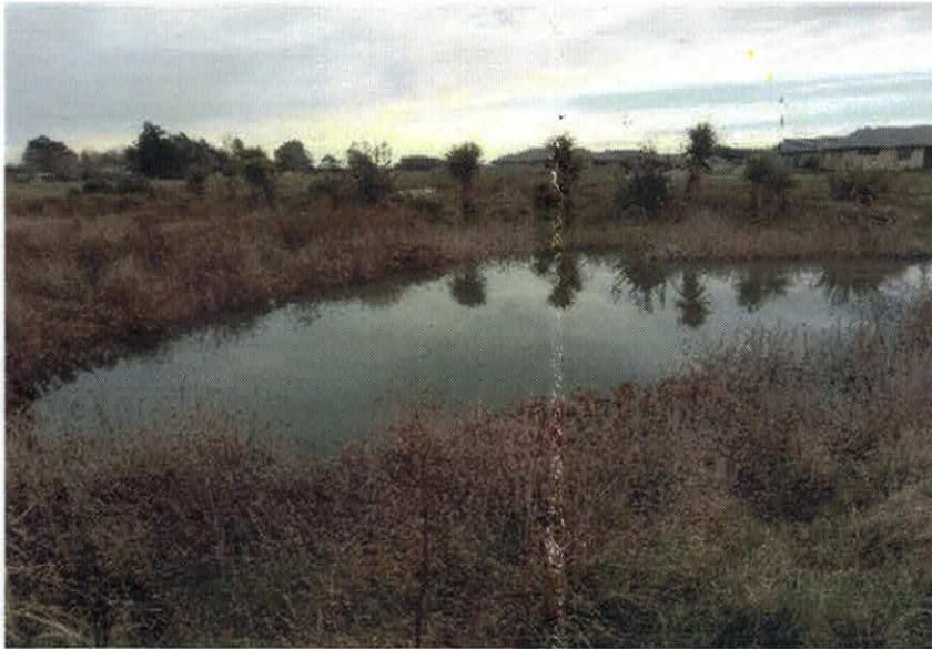
Figure 19 : Wetland providing treatment of stormwater discharge from the northern subdivision of Leeston. Photo taken on the 26 th July 2017
