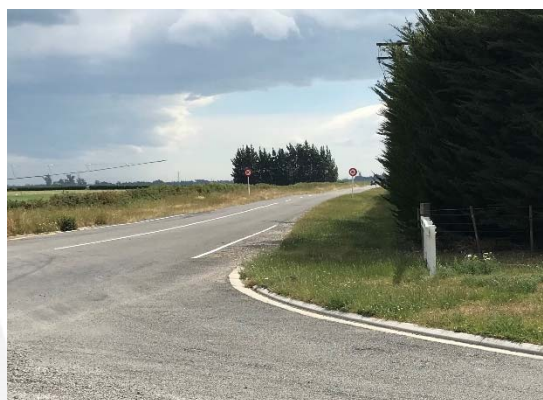
Photographs 3 and 4: Sight Distances to the Left and Right at the Selwyn Road / East Maddisons Road Intersection
