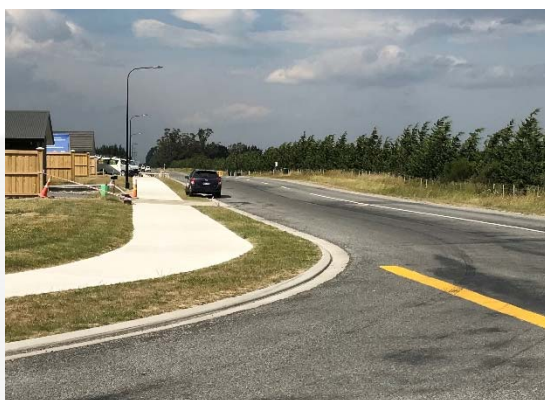
Photographs 3 and 4: Sight Distances to the Left and Right at the Selwyn Road / East Maddisons Road Intersection
