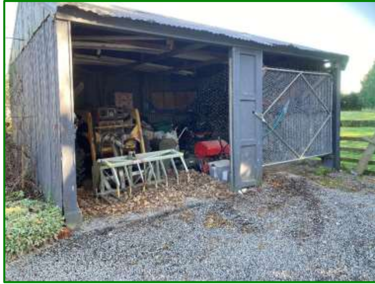
Photo 4: Iron and timber shed storing farm/garden machinery
