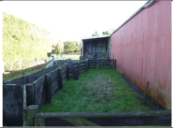
P22: Lot 1 DP 360577 311 Trices Road Sheep race/shute behind implement shed. No below ground structures observed.
