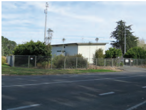
128 Birchs Road / utility
