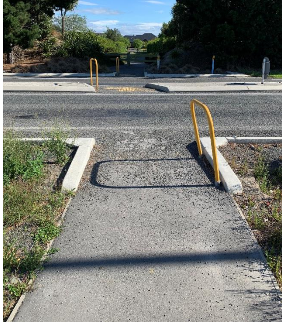
Photograph 3: Pedestrian Refuge Across SH73
