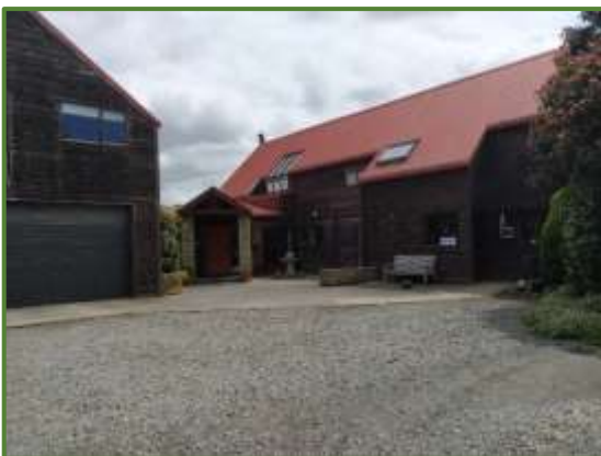
Photo 7 – Dwelling & attached garage
