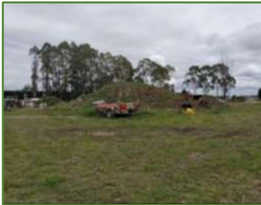
Photo 16 – Stockpile of fill material
