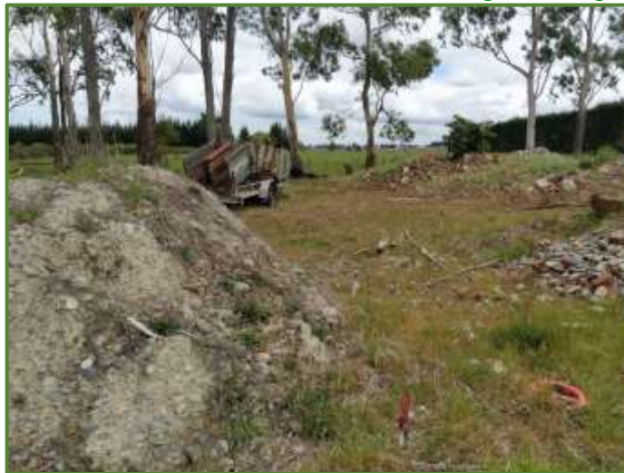
Photo 22 – Stockpiles of fill material
