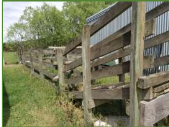
Photo 6 – Loading ramp and holding pen
