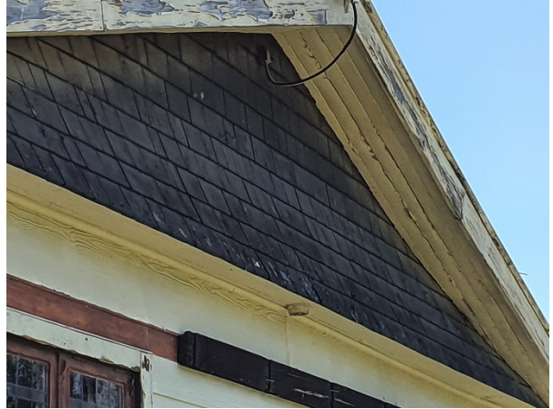
P1 & P2: Dwelling located at Lot 1 26880. Close up shows paint flaking on barge boards.
