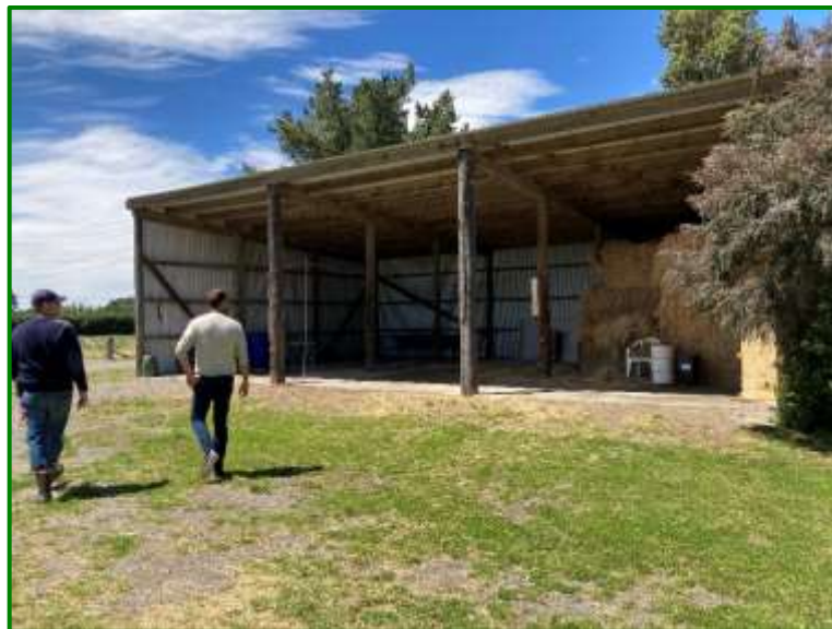
Photo 7: Iron & timber hayshed with concrete floor
