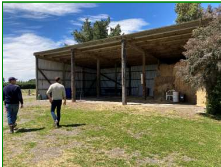
Photo 7: Iron & timber hayshed with concrete floor
