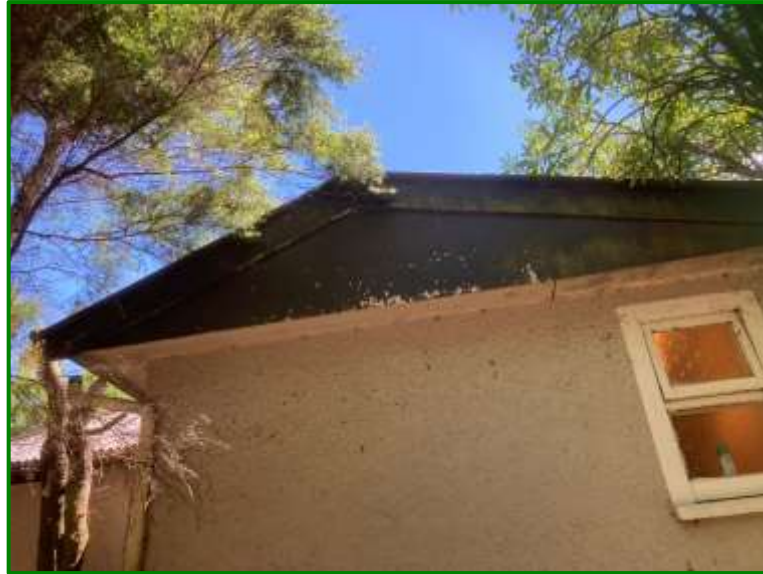
Photo 2: Potential asbestos cement board soffits
