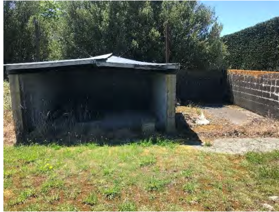
Photo 8: Concrete holding bunkers.
