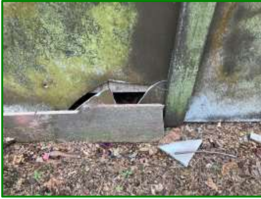
Photo 22: Example of damage to cement board
