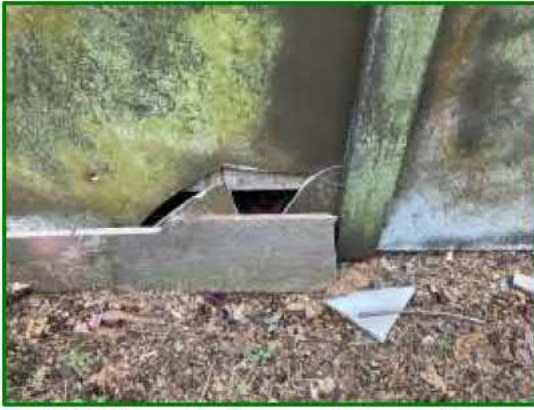
Photo 22: Example of damage to cement board
