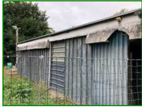
Photo 23: Metal shed with broken cement board
