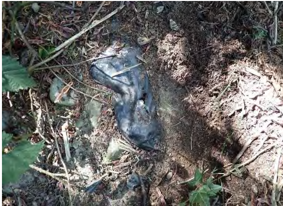
Figure 12. Exposed plastic liner at the soak pit at 15 Two Chain Road.
