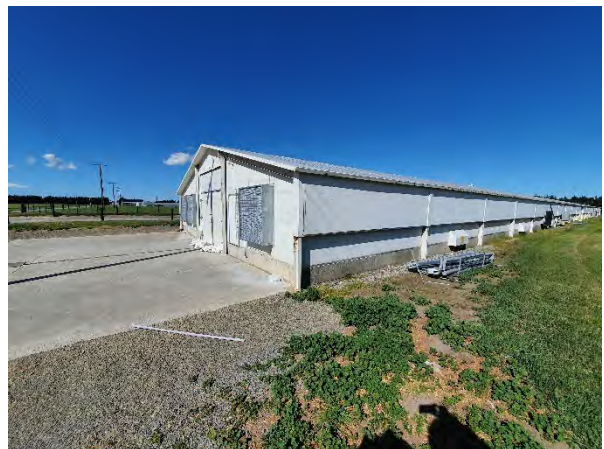
P20: Example of chicken shed clad with "SIP" type cladding.
