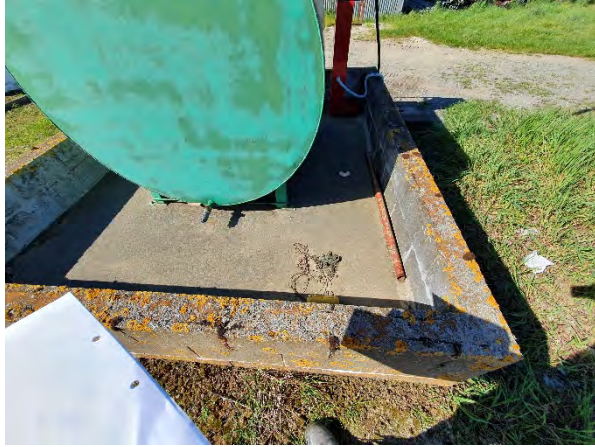
P25: Concrete bund construction and condition. No cracking observed in floor.
