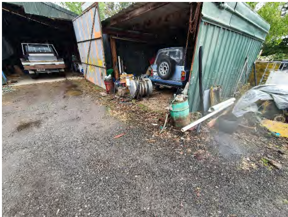
P7: Fuel tank observed in one of the implement sheds. The tank is not fixed, and has no bund.
