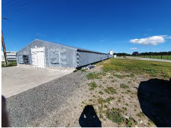
P21: Example of chicken shed clad with profiled metal cladding
