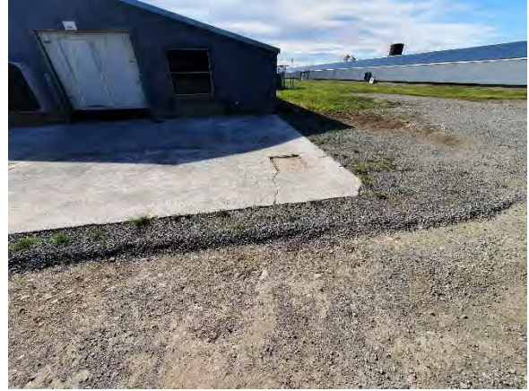
P22: Example of cracking in concrete pad at end of chicken shed.
