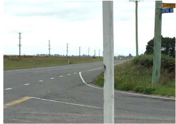
Photographs 3 and 4: Sight Distances along State Highway 73 from Creyke Road at 5.5m Back from Traffic Lane Showing Effect of Shelterbelt
