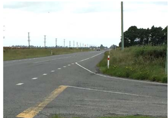
Photographs 5 and 6: Sight Distances along State Highway 73 from Creyke Road at 3.5m Back from Traffic Lane Showing Excellent Distances
