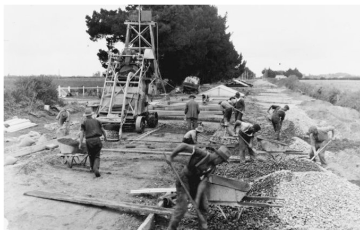
Templeton-Rolleston section of SH1 being built, c. 1930. Source: PAColl-6181-56, Alexander Turnbull Library, Wellington.
