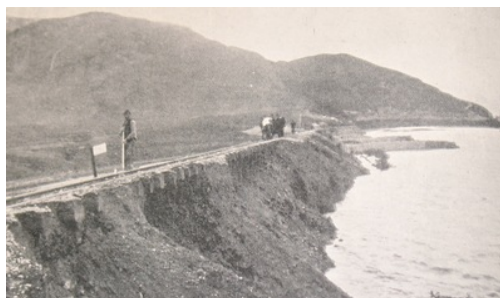
Waimakariri River in flood; a washout on the railway line near Cass, 16 November 1926. Source: Selwyn Kete.
