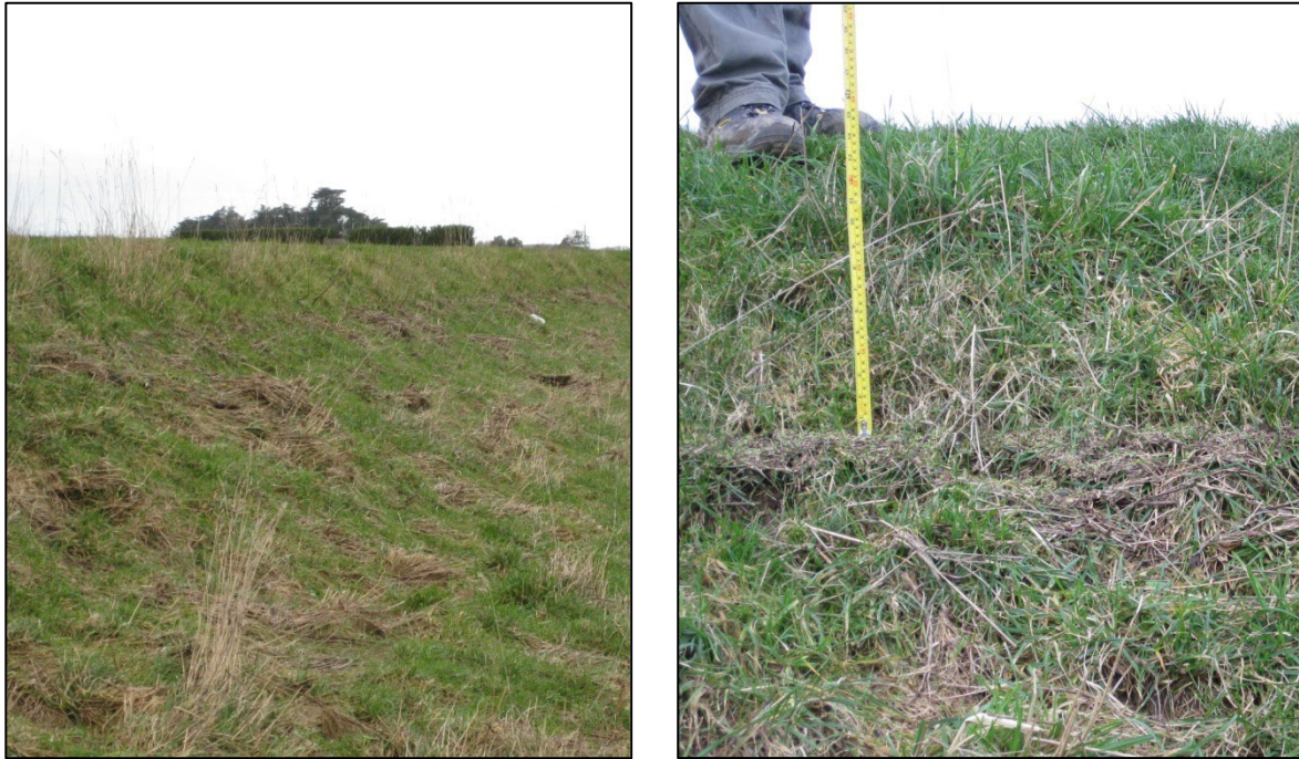
Figure 3-5: Flood/debris marks on stopbank downstream of Coes Ford (4 August 2008)
