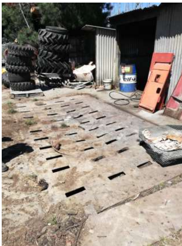
Photograph 8: Tractor wash / 3 stage interceptor (Area 3)
