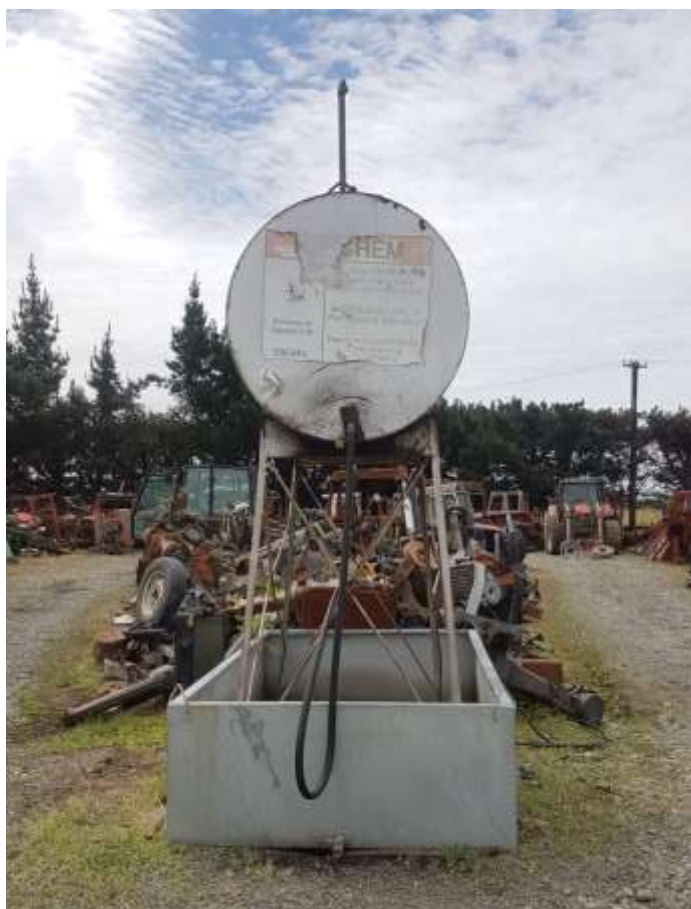
Photograph 13: 2000L bunded diesel tank (Area 3)
