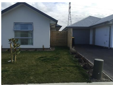
Figure 1 - the photo shows a garage positioned 1m off the side boundary but with the eaves of the adjacent buildings almost touching. By having a concrete block wall for the garage on the boundary and pushing the house on the left over 1m, a two-metre wide gap would be created and would provide more useable space and allow more light into each dwelling. The 1m wide yards either side of a 1.8-2.0m high close board timber fence is considered inefficient use of land and could be improved.
