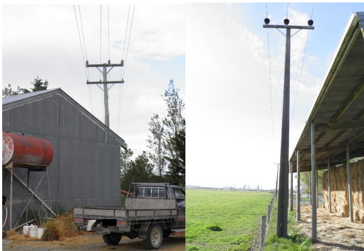
Figure 9: Underbuild and encroachment on Orion's high voltage network.
