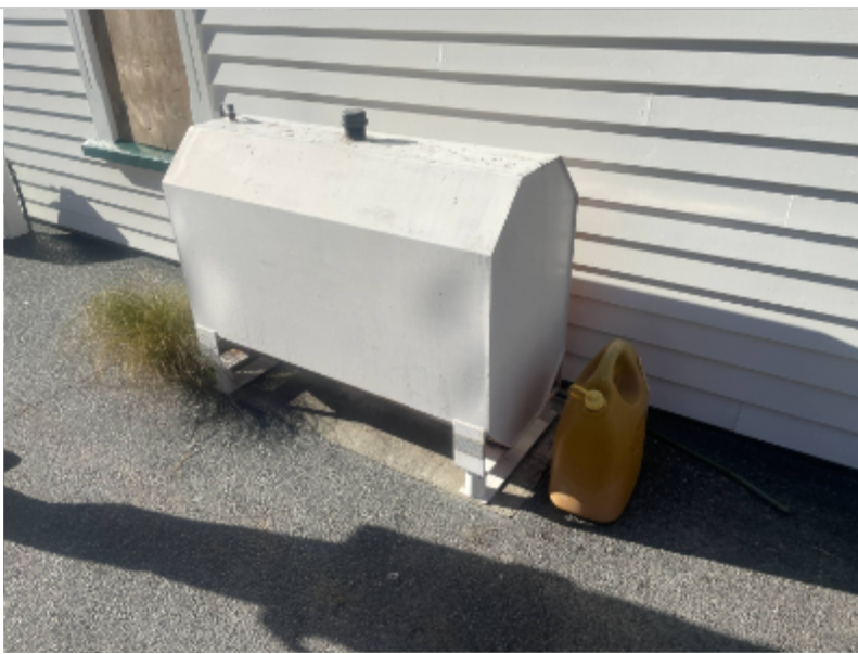
480L Above Ground Diesel Tank - 966 Selwyn Road
