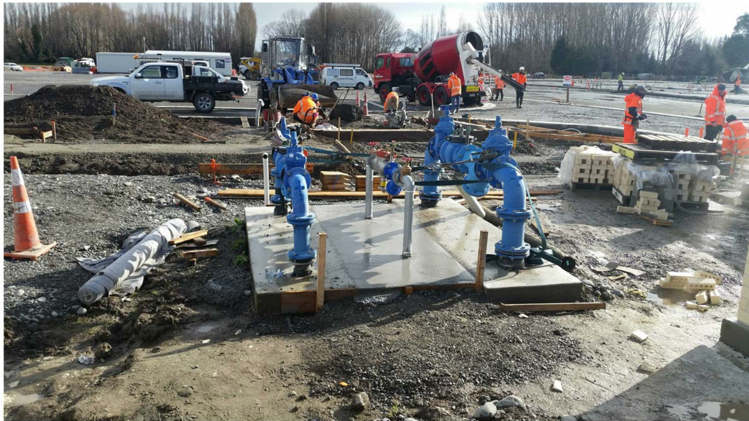
7 Backflow Preventer Enclosure - Images Not To Scale
