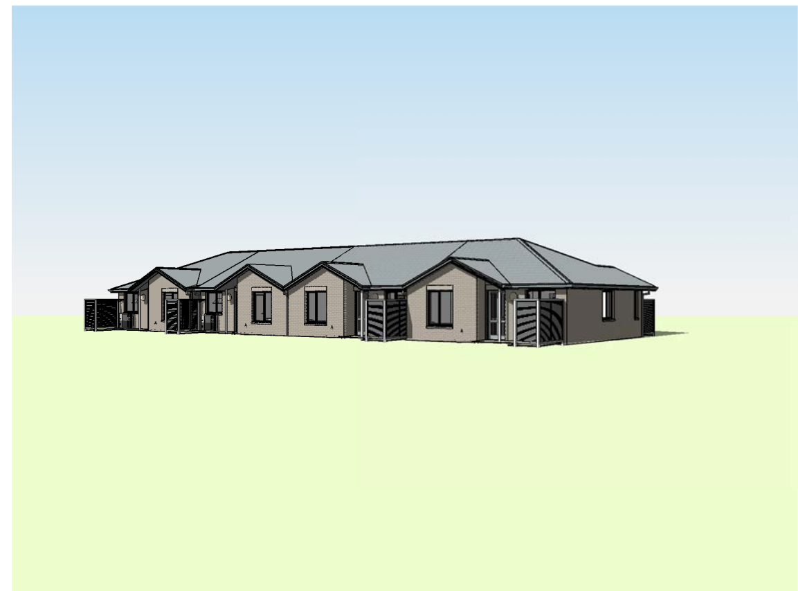
8 COTTAGE (NO GARAGES) 4 BLOCK - REAR VIEW
