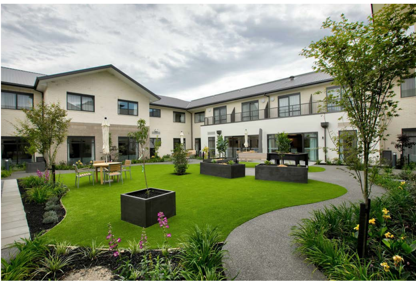
Casebrook Main Building internal courtyard
