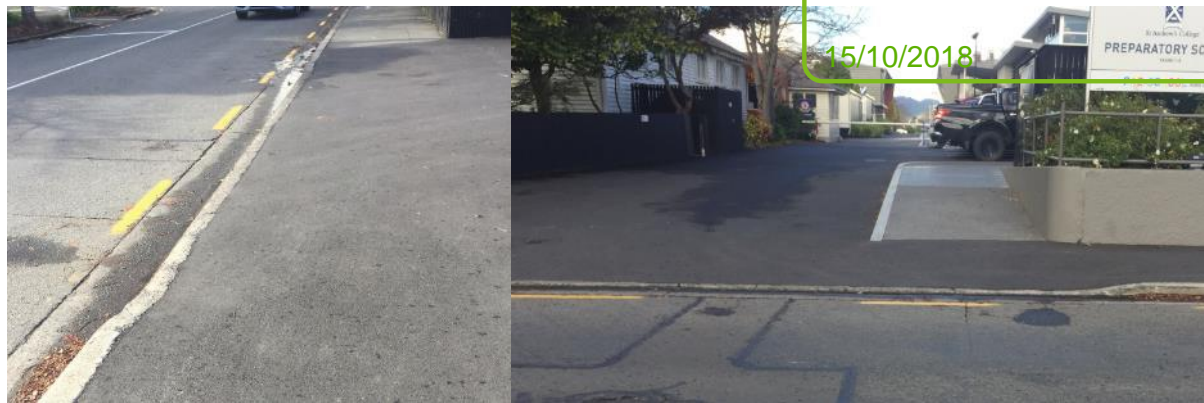
Figure 2-5: Wide vehicle crossing and pedestrian ramp
