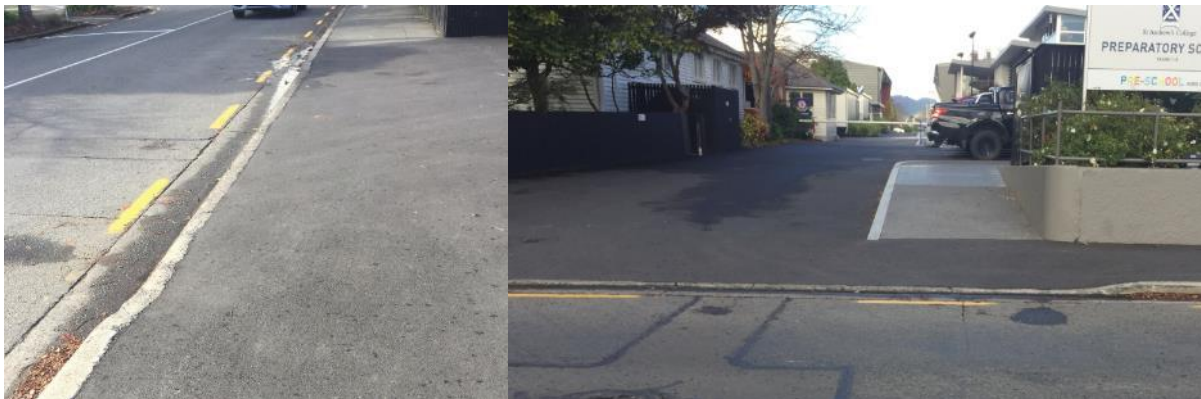
Figure 3-1: Wide vehicle crossing and pedestrian ramp
