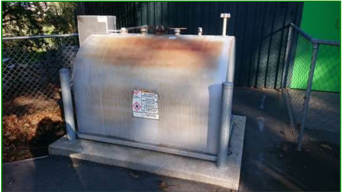
Photo 1 - Tank exterior appears in good condition, concrete pad appears clean with no evidence of spills or leaks
