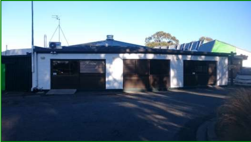
Photo 3 - Exterior of building: painted concrete block, timber and iron
