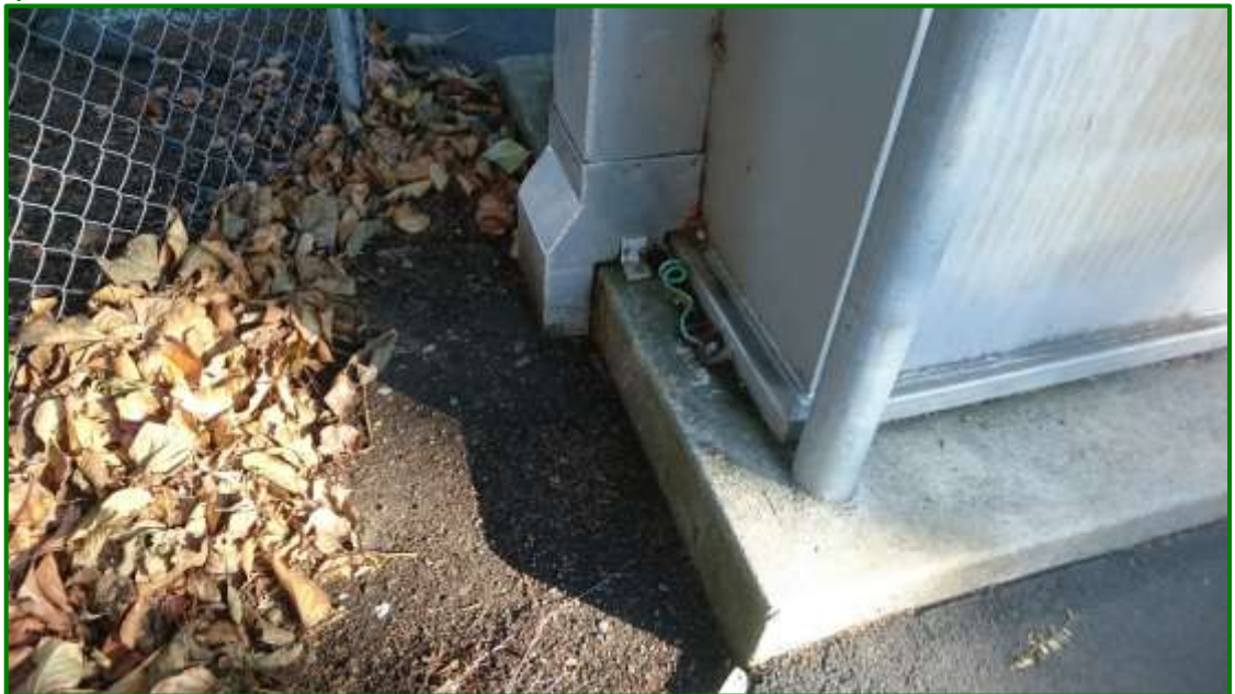
Photo 2 - Bare earth at end of tank, no evidence of spills or leaks
