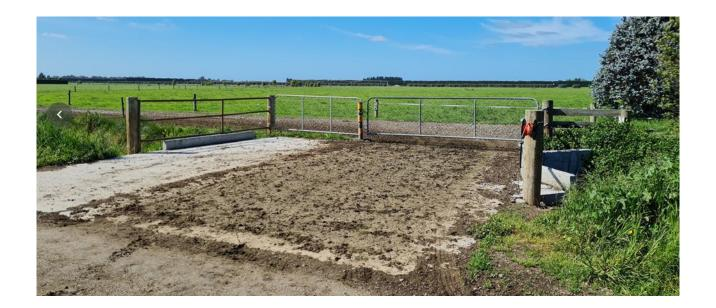
The vehicle access for Stages A and B off Buckleys Road appears to be constructed to Council standards: Diagram E10.D, except that there are no sealed tapers. Therefore, it does not meet Rule 4.5.1.2 (Any vehicle accessway is formed to the relevant design and formation standards set out in Appendix E10.2), and consent is required as a Discretionary Activity under Rule 4.5.4: Vehicle Accessways and Vehicle Crossings.
