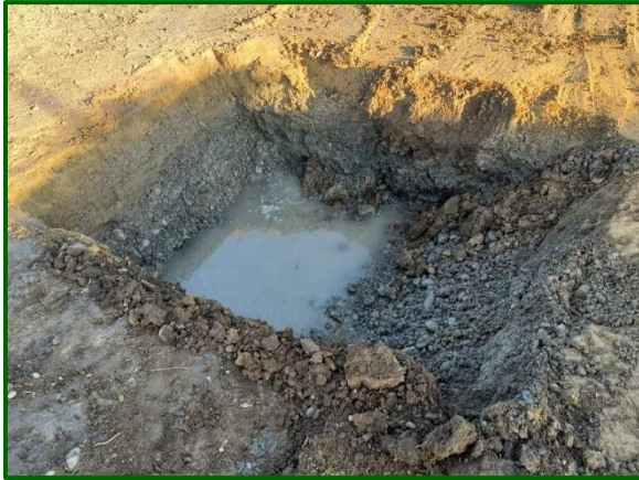
Photo 8 – Deeper excavations required in yard
