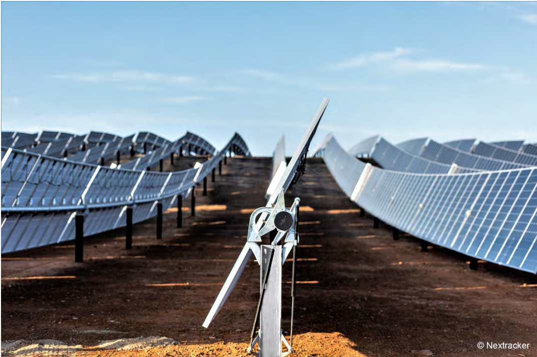
Figure 2: Typical solar Single Axis Tracking PV table configuration.
