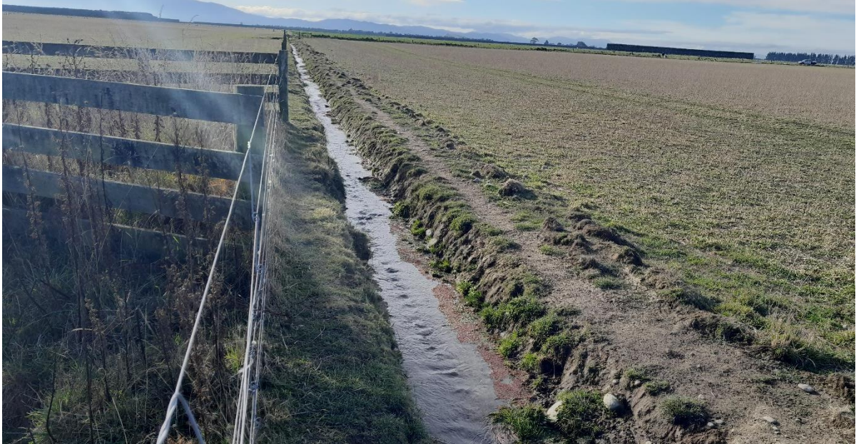
Figure 8: The water race that bisects the site showing shallow surface water, homogenous run habitat and no channel shade.
