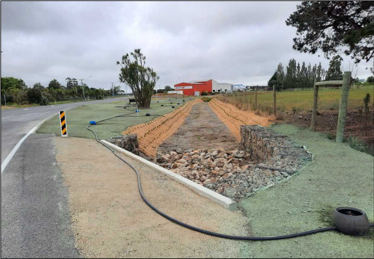
Photo 5: Upgraded Culvert (southern side) and Volckman Drain. Looking east from Station Street towards Volckman Road.
