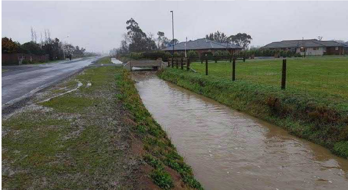
Image 2: Upgraded Manse Road Drain in Flood
