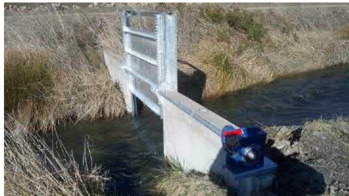
Figure 9 - Kowai Gate control mechanism accessed from the side
