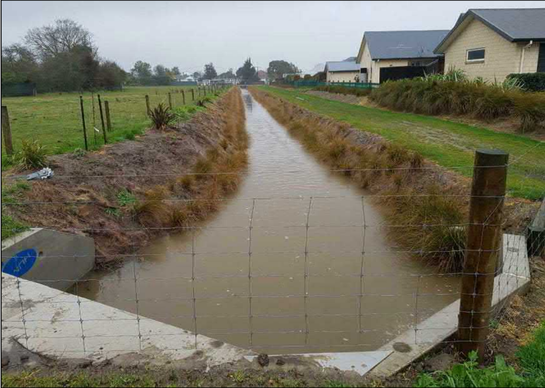
Photo 1: Upgraded Ellesmere Hospital Drain in Flood. Looking west from Manse Road towards Cunningham Street (Ellesmere Hospital – left).
