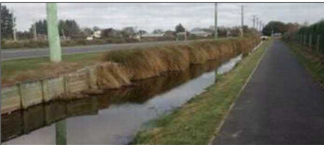
Photo 2: Widening of High Street Drain.
