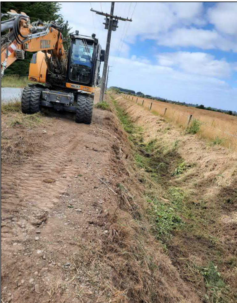
Photo 10: Volckman Road Drain - After Maintenance
