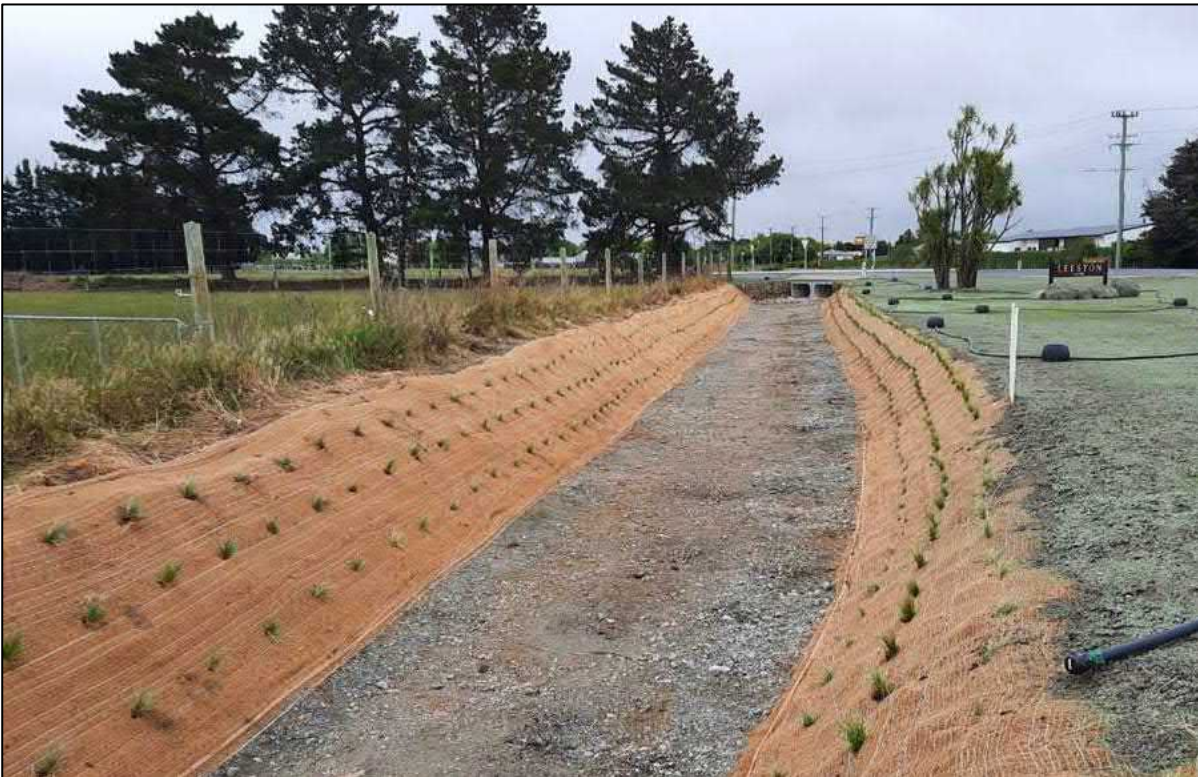
Photo 6: Upgraded Volckman Drain. Looking west from Volckman Road towards Leeston Road/High Street.
