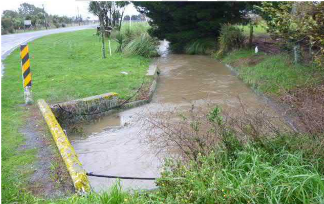
Image 3: High Street Culvert Outlet in Flood – June 2013
