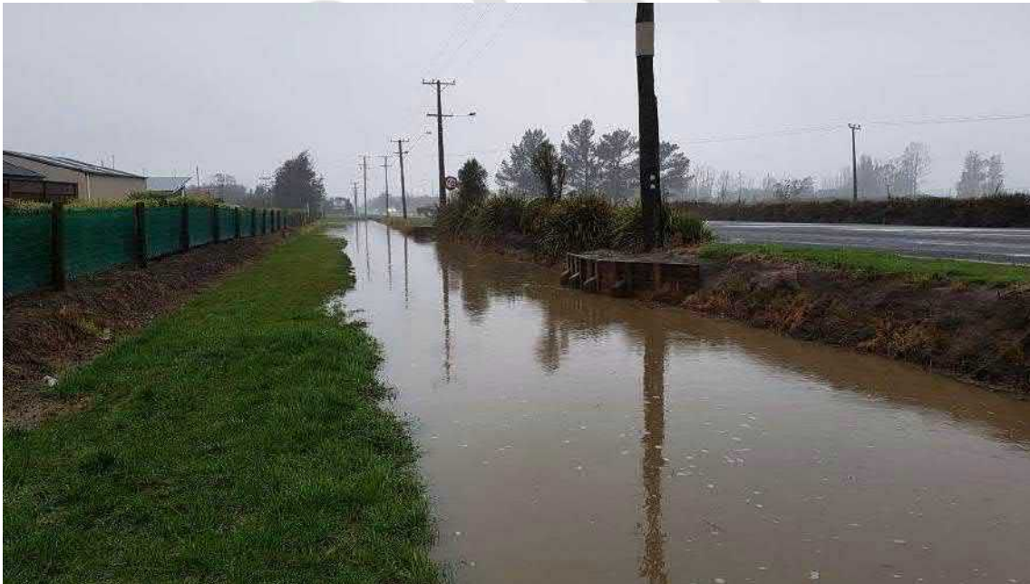
Image 1: Upgraded High Street Drain in Flood
