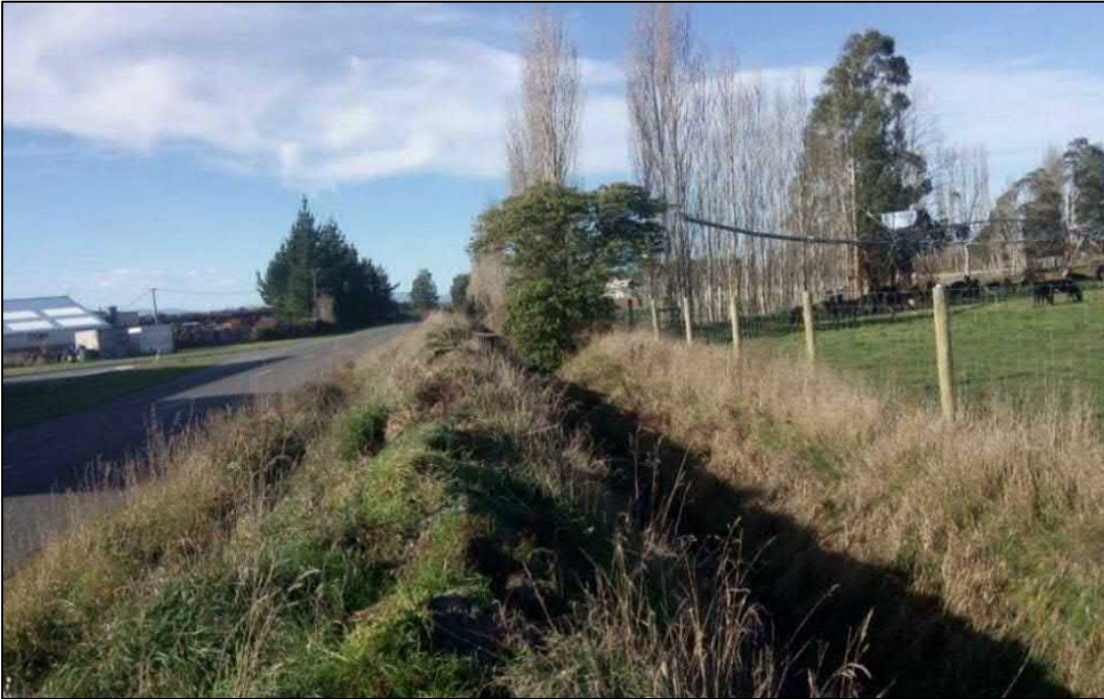
Photo 7: Volckman Road Drain - Before Maintenance
