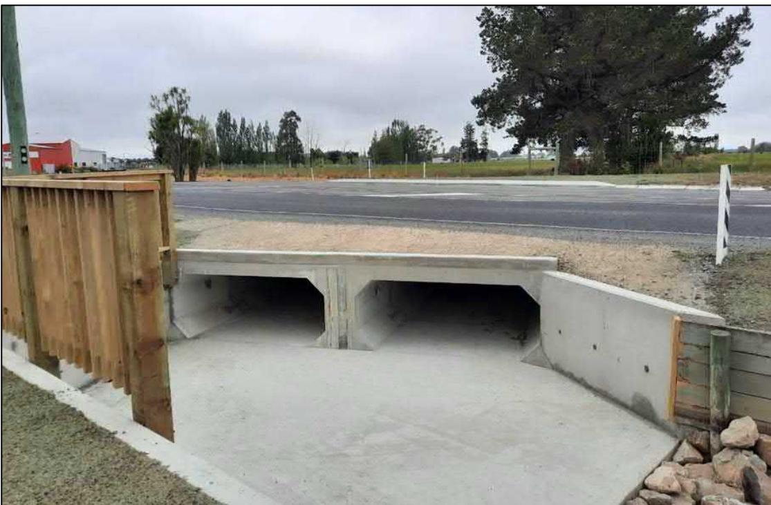
Photo 4: New culverts under High Street (northern side) Looking south.
