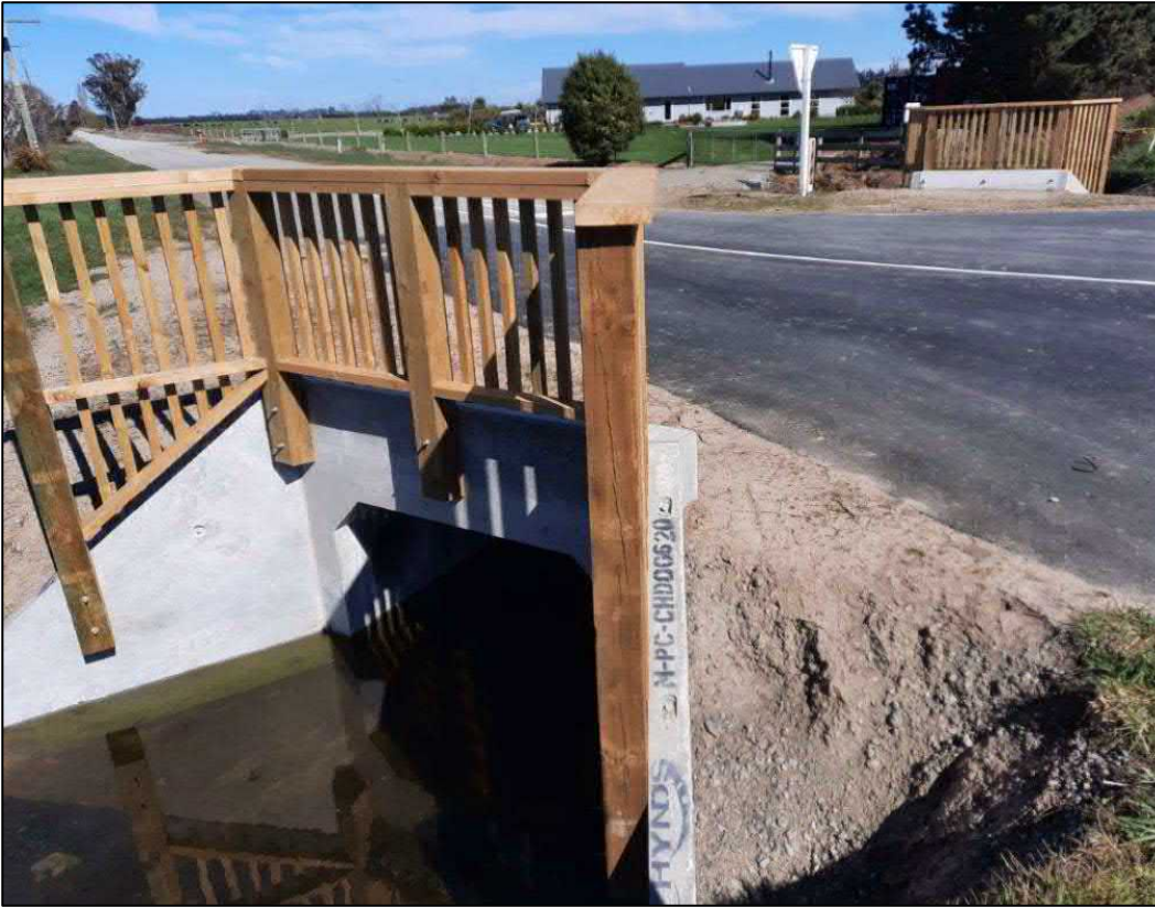
Photo 11: Volckman Road Drain - Beethams Road - upgraded culvert. Looking West at intersection of Tramway Reserve Road and Beethams Road.
