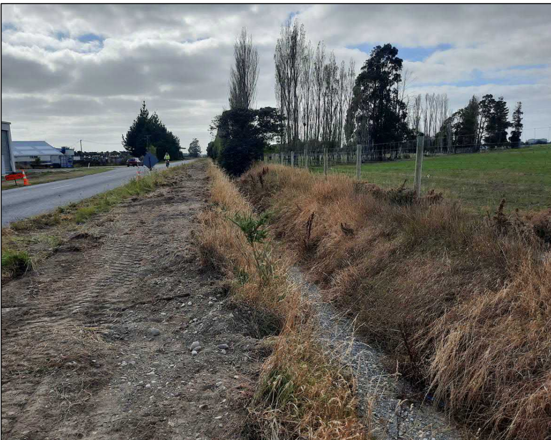
Photo 8: Volckman Road Drain - After Maintenance
