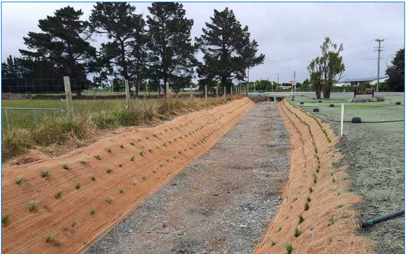
Leeston Stormwater Flood Bypass Scheme – Completed Stage 3 Works
