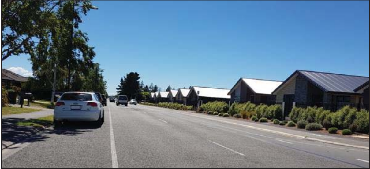
Figure 3.8 Lowes Road cross section looking east toward site, with the footpath on the left side and shared path on the right
