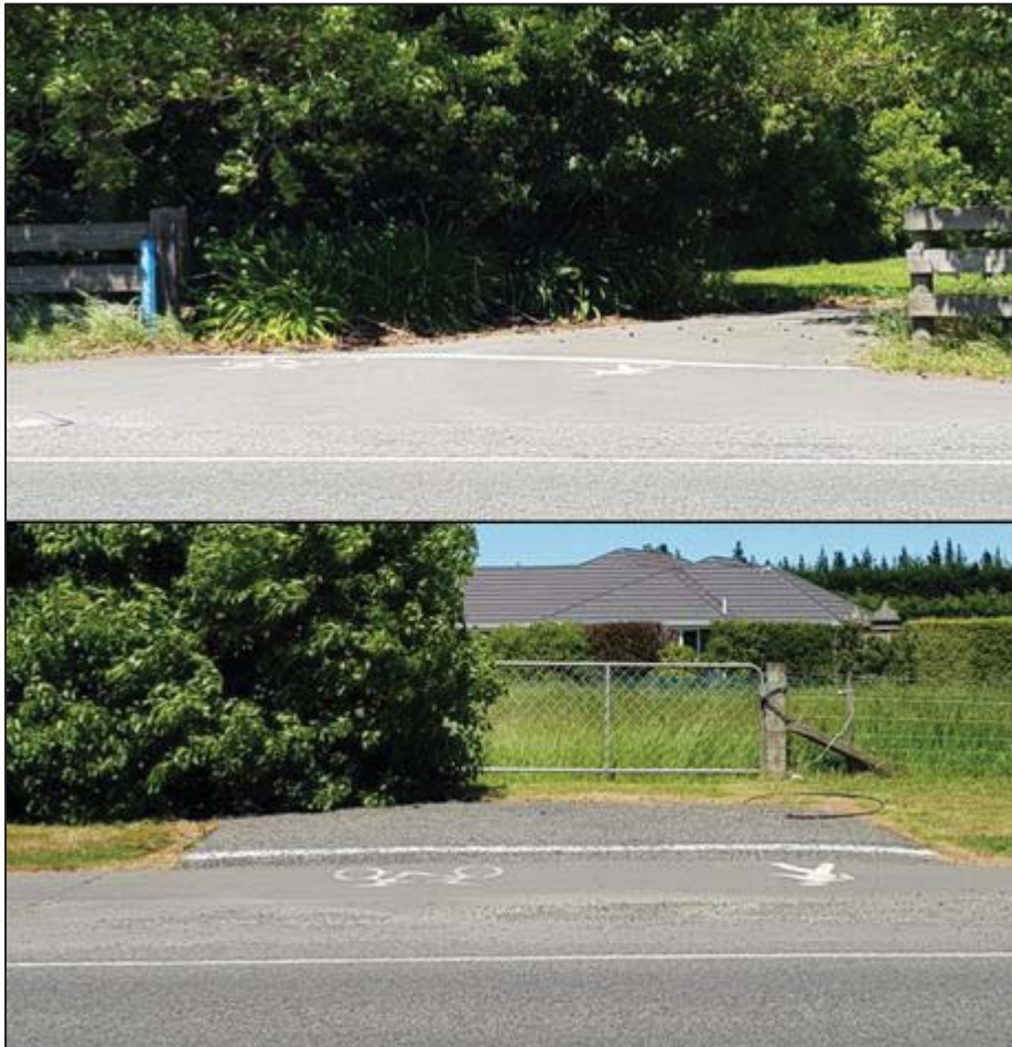
Figure 3.5 Shared path markings on Lincoln Rolleston Road
