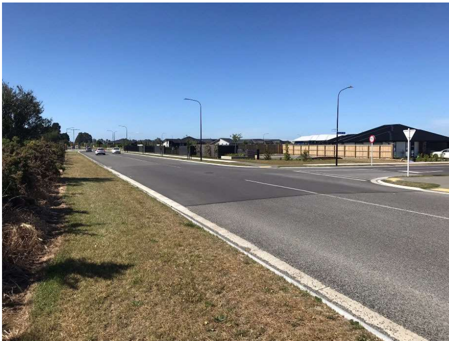
Figure 3-1: Goulds Road looking North on Site Frontage
