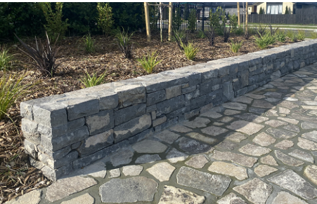
Low feature walls with oxford grey basalt veneer. Used to frame key entry points into the development. Opportunity to integrate seating into the design. The basalt veneer will tie into materiality of walls existing in the surrounding Faringdon development.
