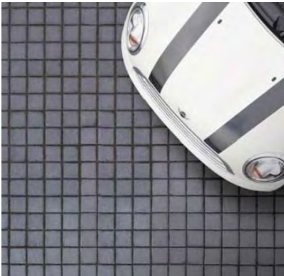
Firth precast concrete modular paving ('Holland' modules) to key pedestrian entry points into the site (flush with adjacent concrete surface).
