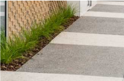
Two tones of concrete to define key areas and entry point and create surface/texture contrast with asphalt roading.
